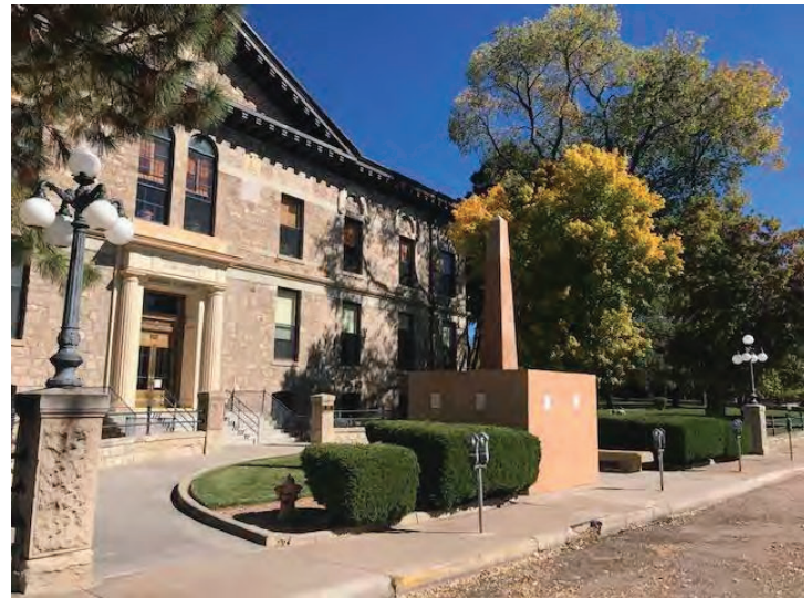
Carson Monument in 2021—boarded up to prevent graffiti/destruction (photo—D. Swanson 2021)
